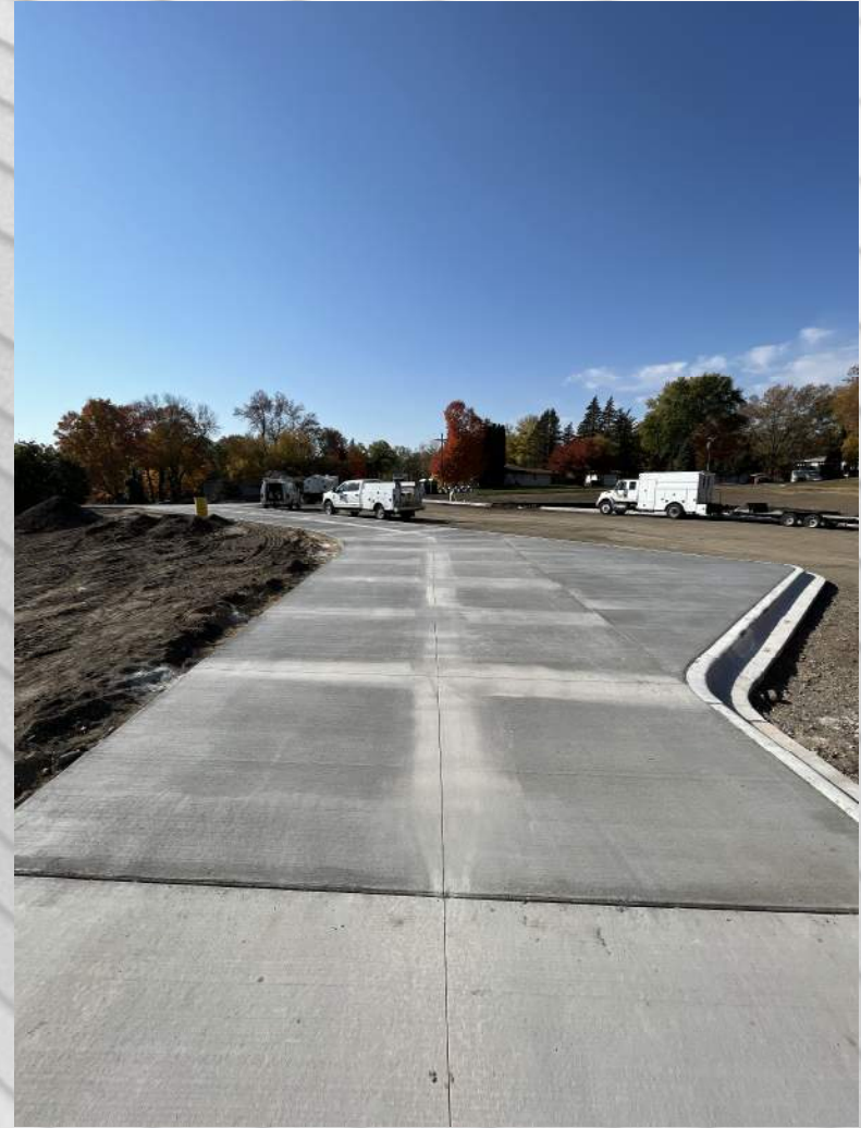
Remainder of sidewalk poured
