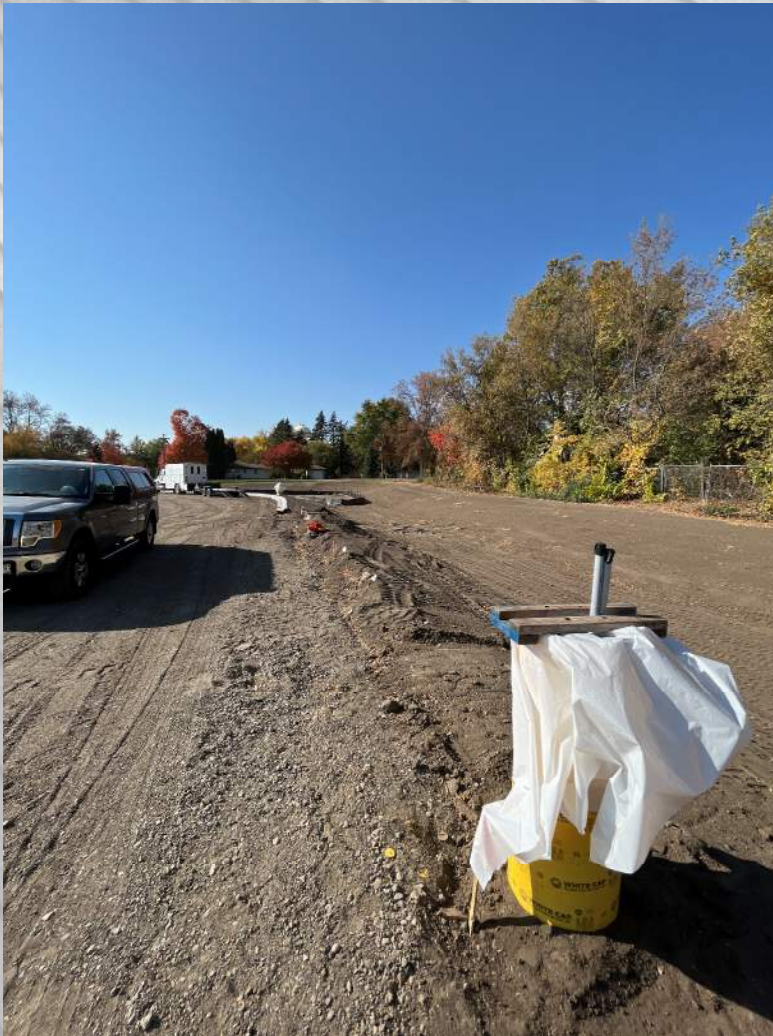
Light bases formed and ready for concrete
