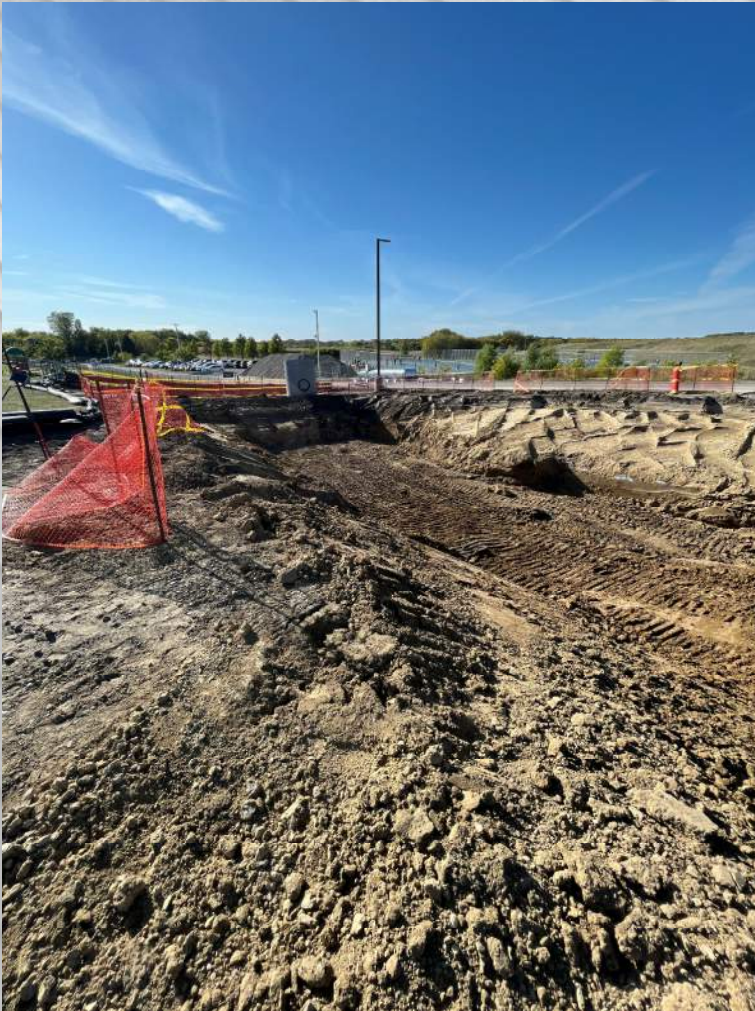
Excavations for underground storage system
