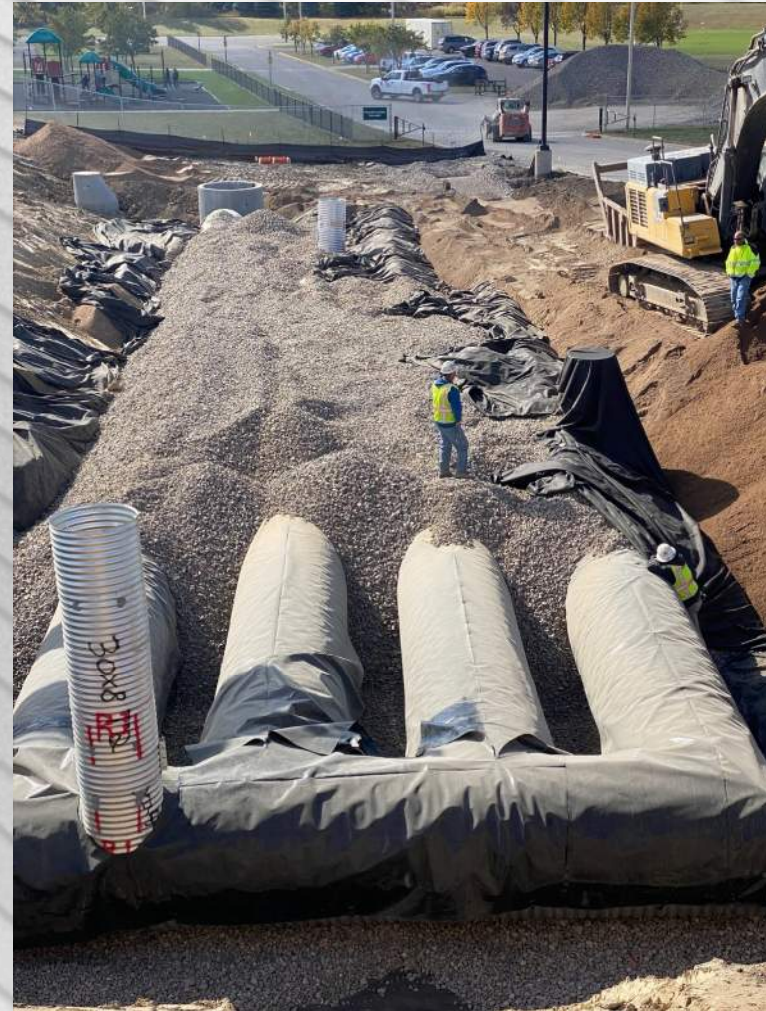
Underground storage system installed and backfill underway
