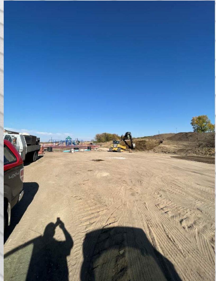
Storm sewer complete and backfilled
