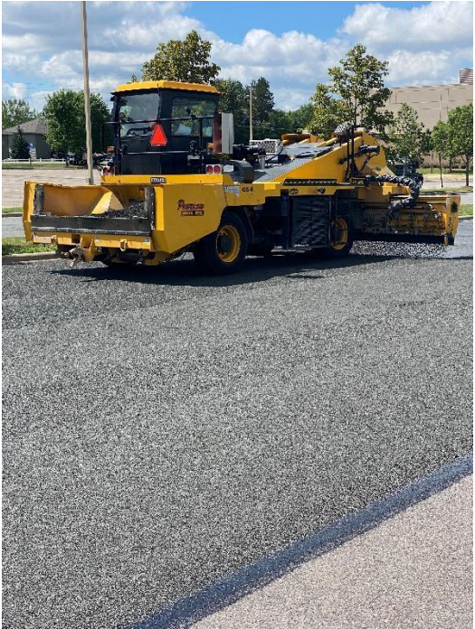
Seal and rock chip at the HS, RCC and bus garage
