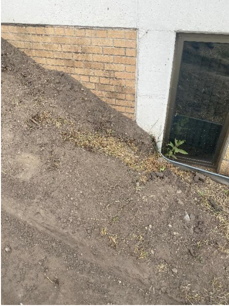
Trench at the MS to divert water from entering the building.
