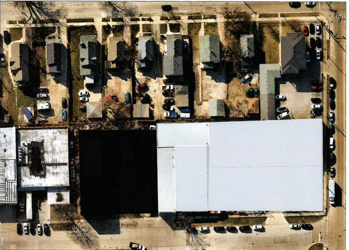
01 AERIAL PHOTOGRAPH - SITE W FUTURE STORAGE FACILITY NOTES
