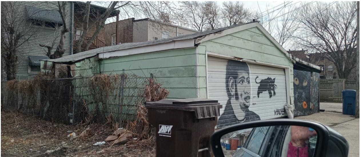
Rear garage showing severe dilapidation and breach of north facing wall, making it subject to the elements, including water intrusion.
