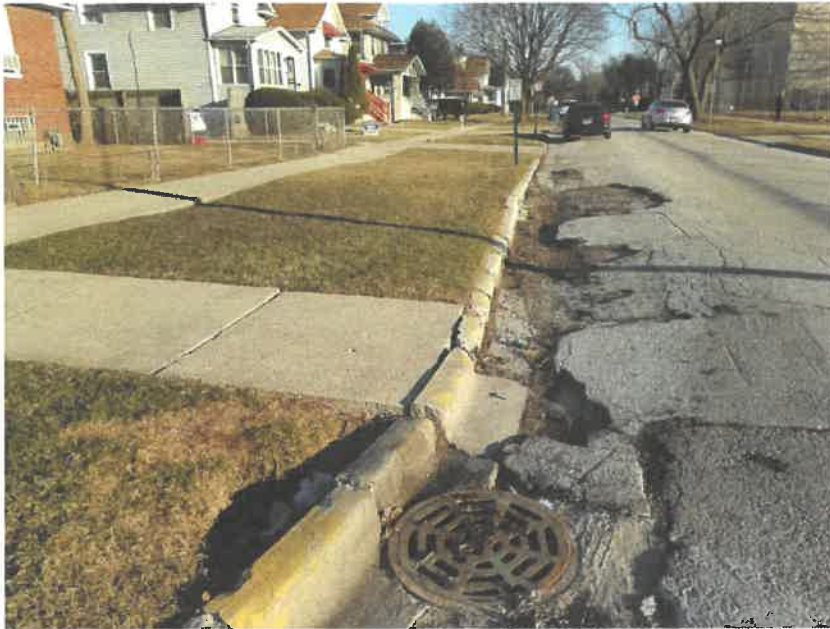
600 BLOCK OF 2 ND AVENUE LOOKING NORTH (BEFORE CONSTRUCTION)
