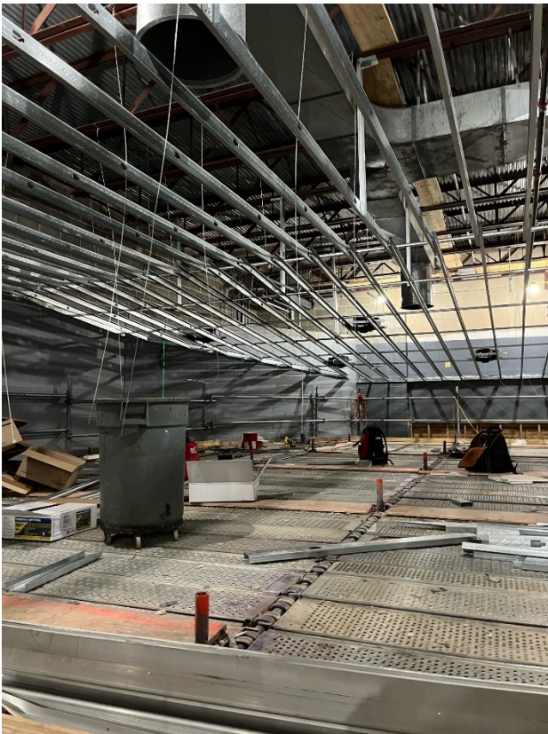
Auditorium Ceiling Framing
