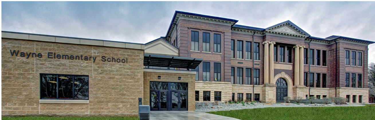
Fig. 3.2.2: Exterior front facade showing 1923 Building and 2010 Addition, 2013
