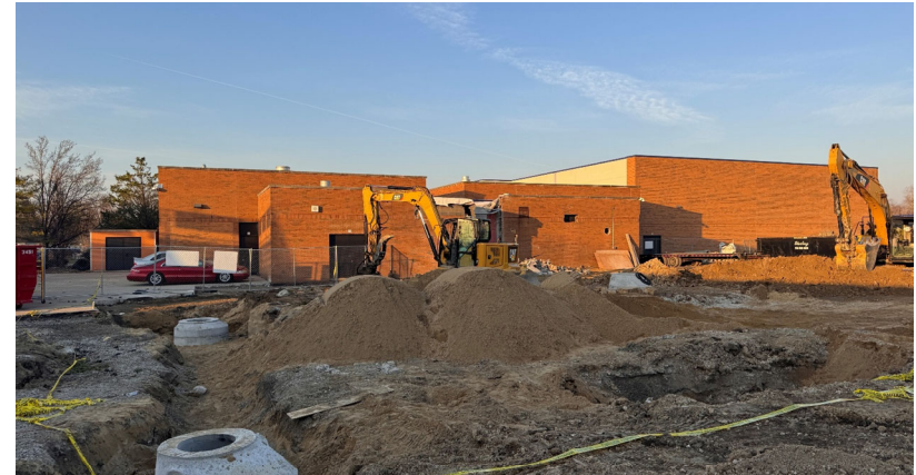
Farmington HS – Site Utilities
