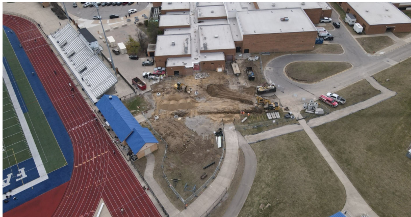
Farmington HS – Demolition
