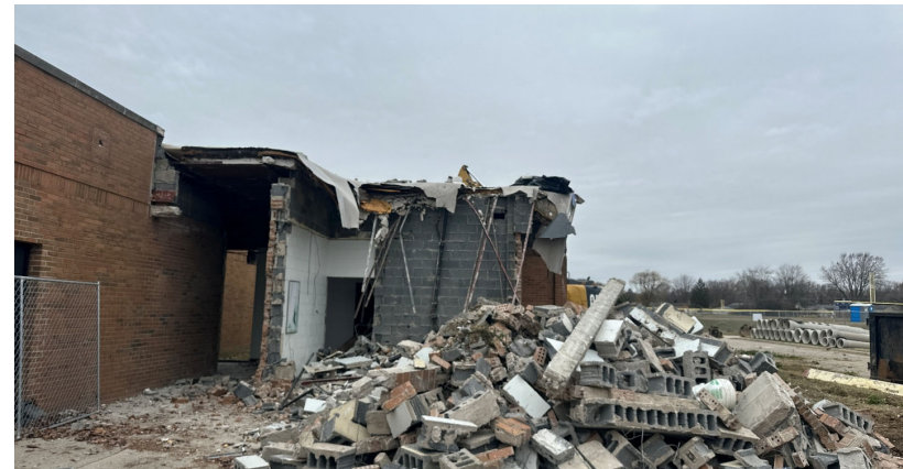
Farmington HS – Demolition
