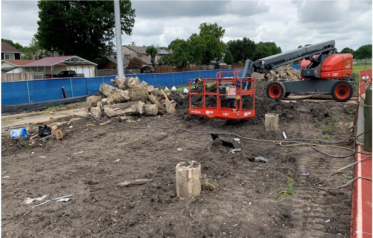
North Garland HS – Demolition
