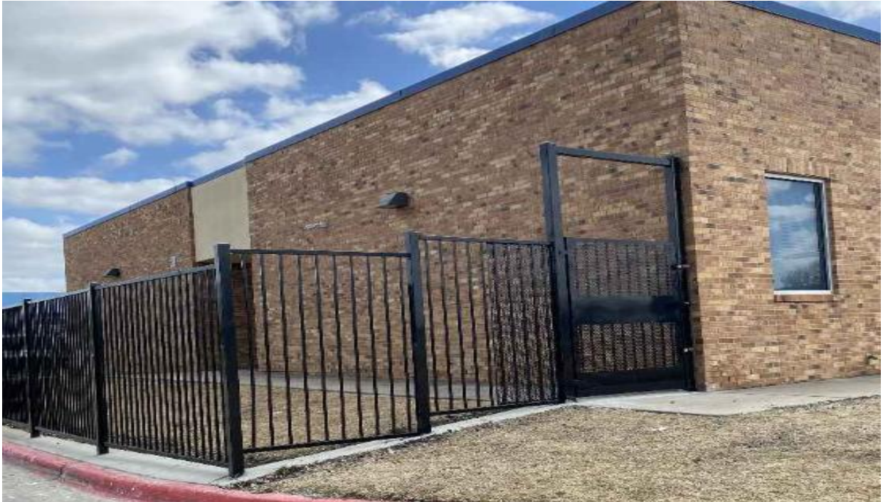
Fence and pedestrian gate at Bradfield ES
