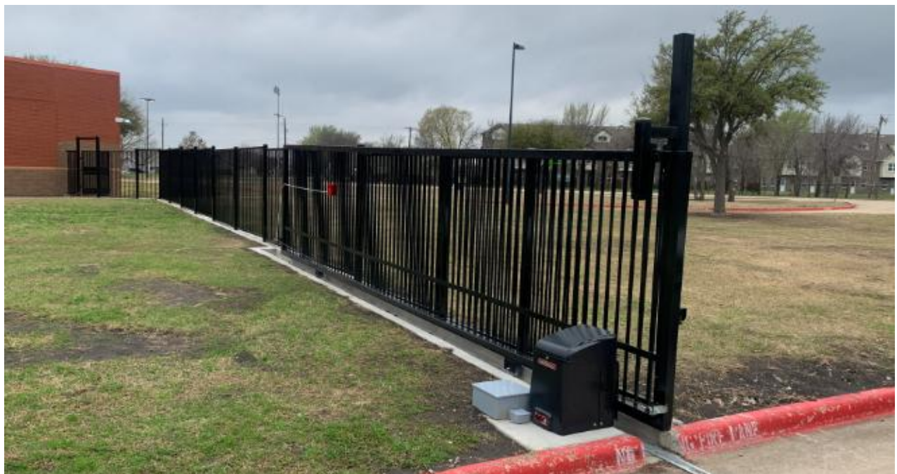
Vehicle gate and fence at Armstrong ES
