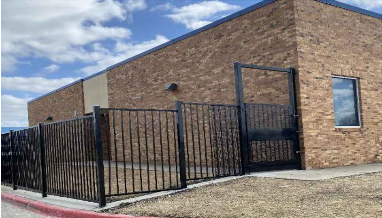
Fence and pedestrian gate at Bradfield ES
