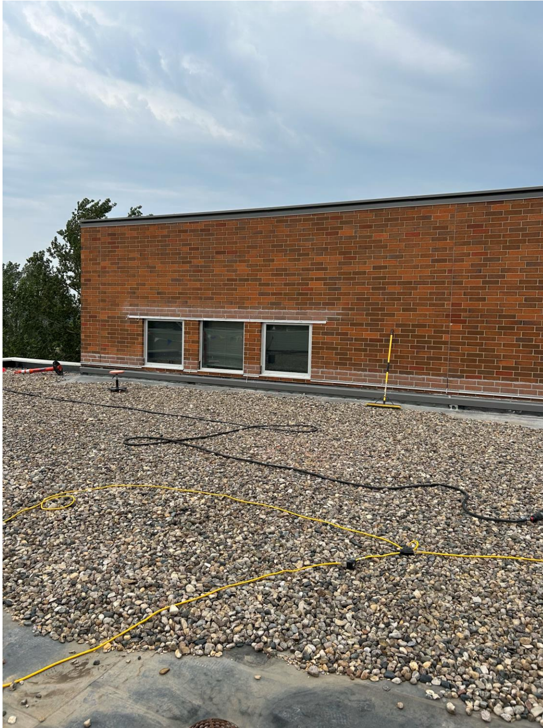
Completed Through Wall Flashing (Green Area)
