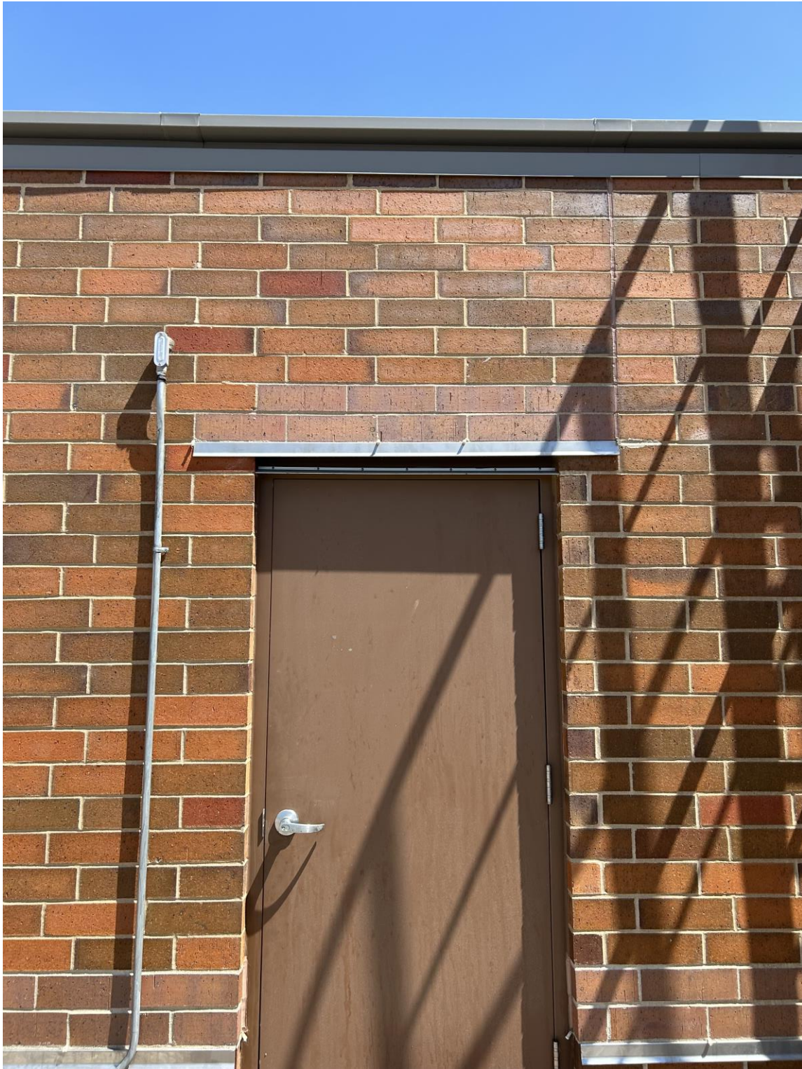
Through Wall Flashing Complete Above Door. New Weeps & Regelet (Blue Area)
