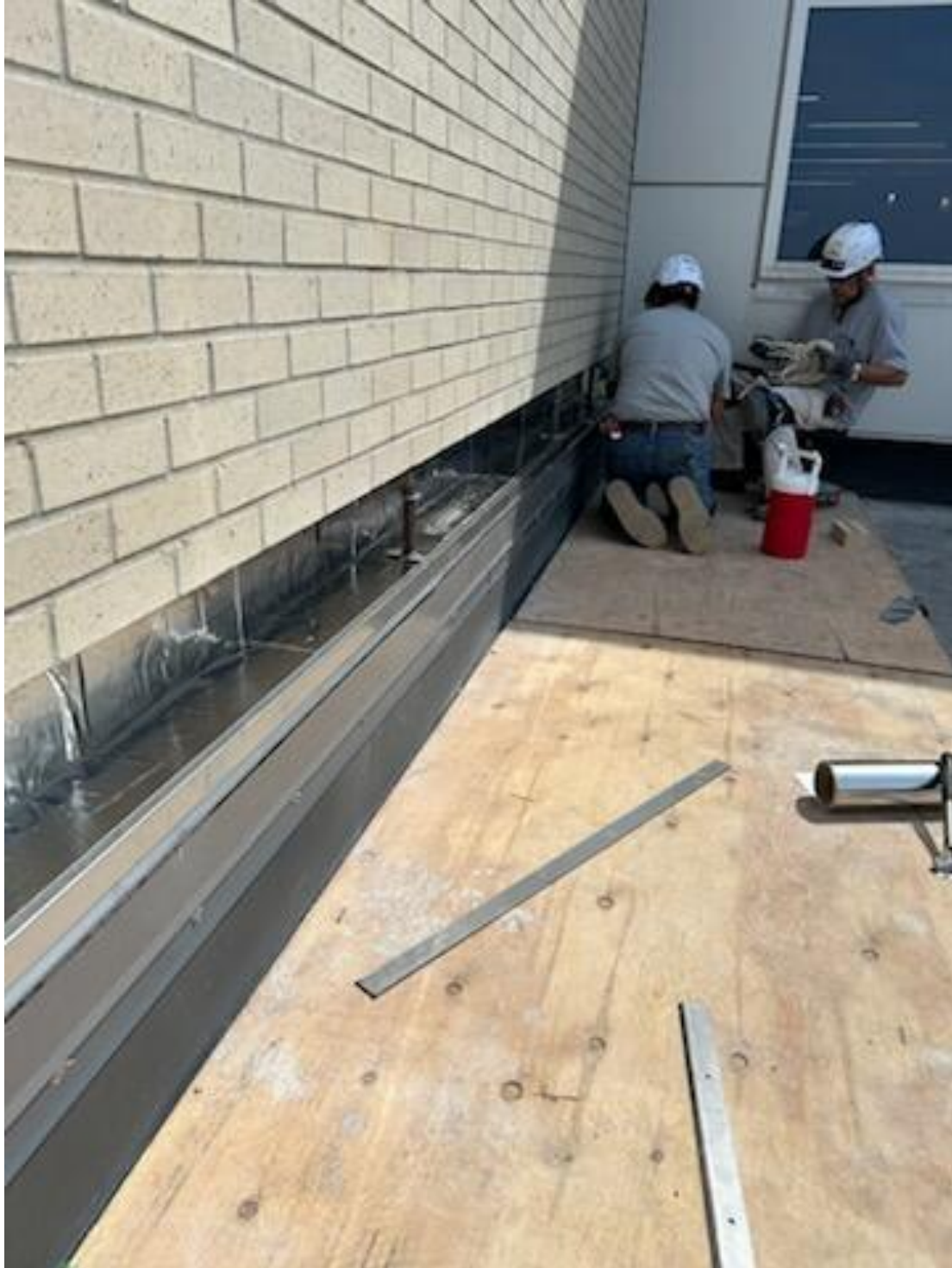
Plywood Protection noted on top of Existing Roofing Membrane
