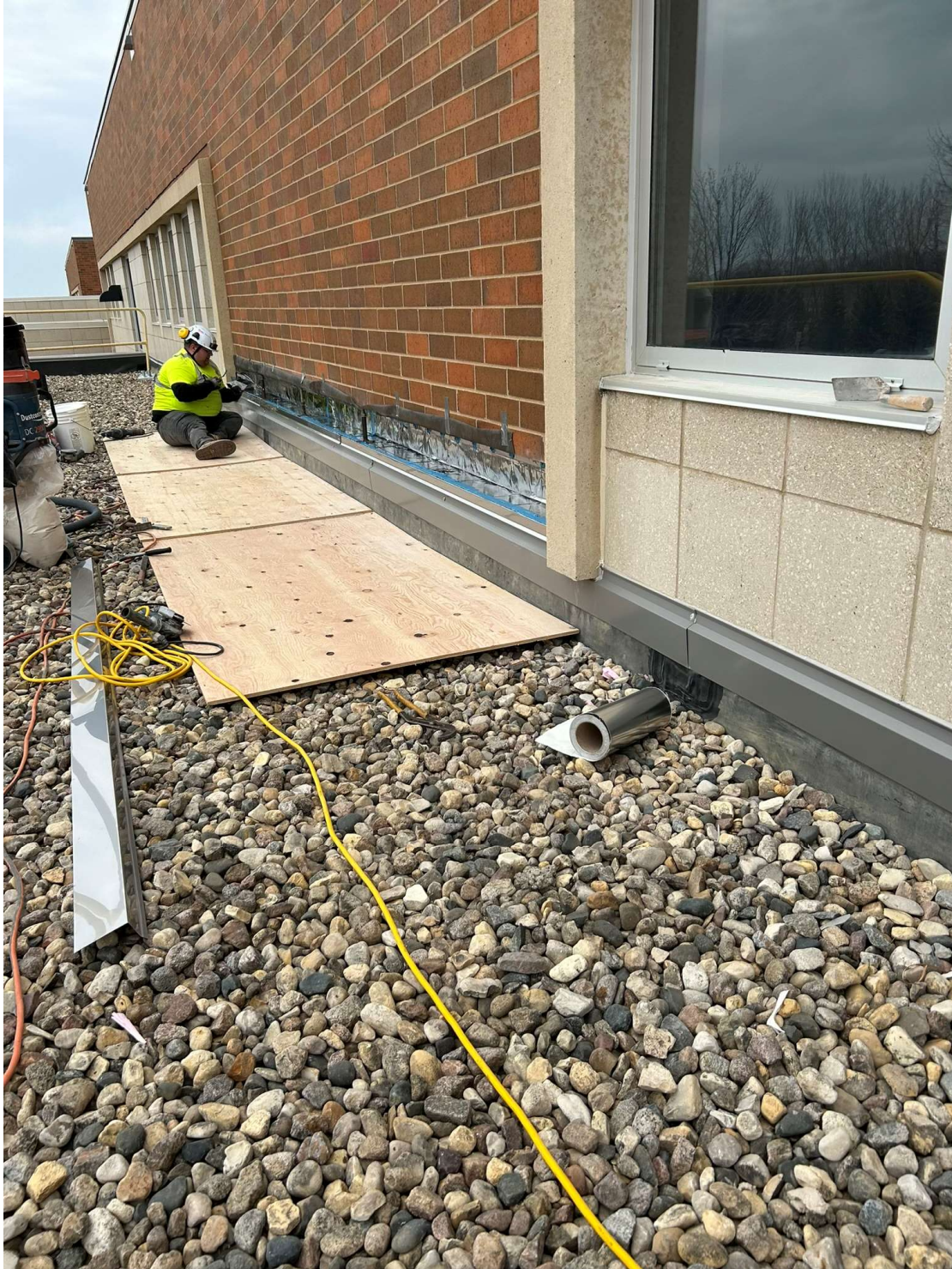
Through wall flashing installation in progress
