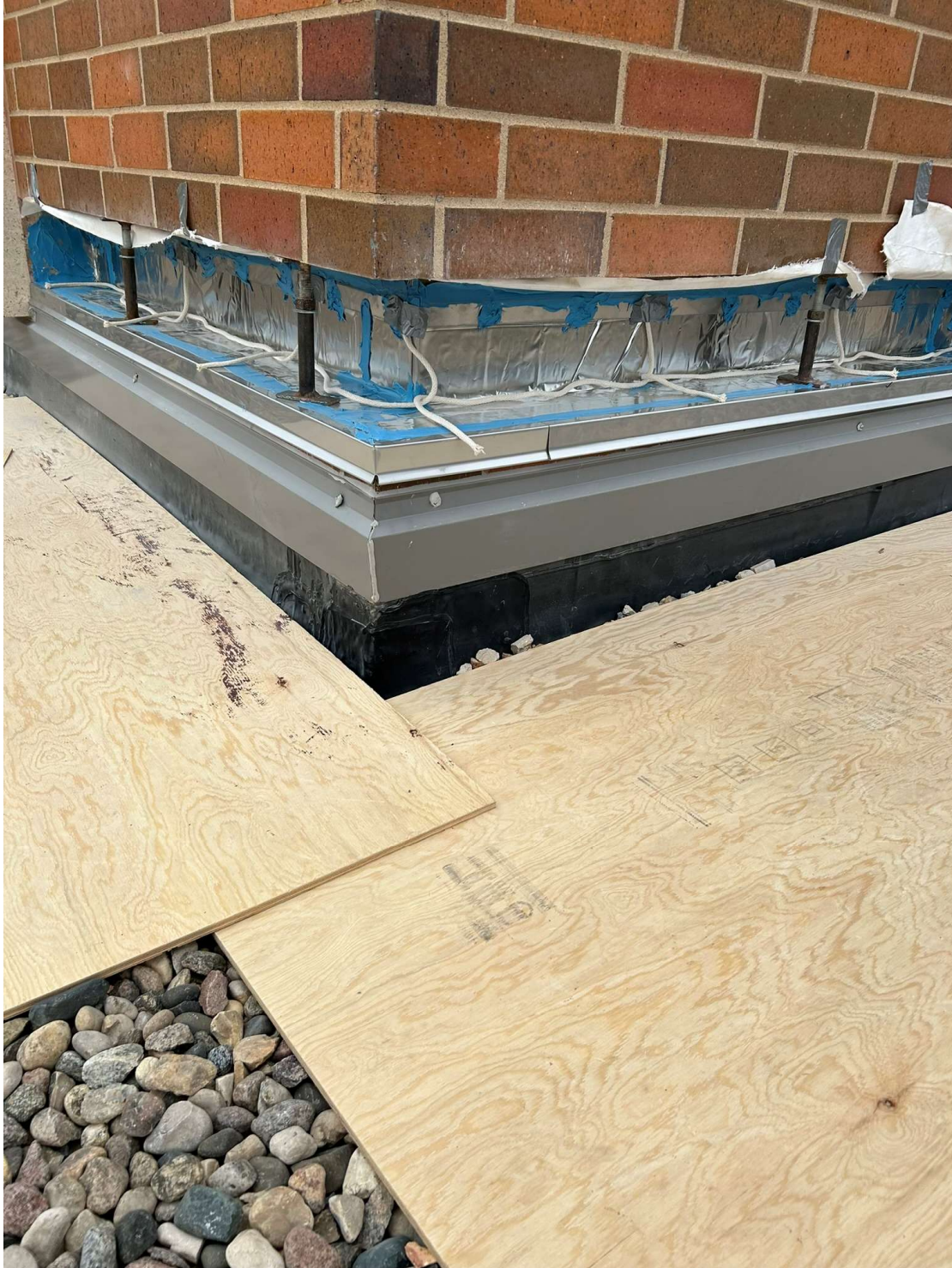
Completed through wall flashing detail ready for brick installation
