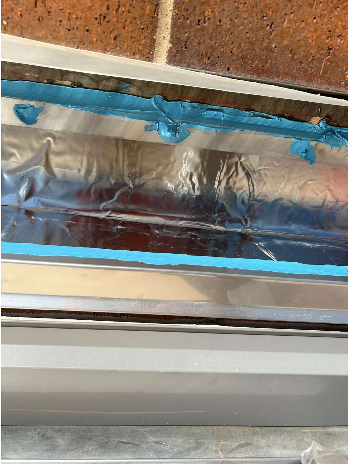
New through wall flashing detail
