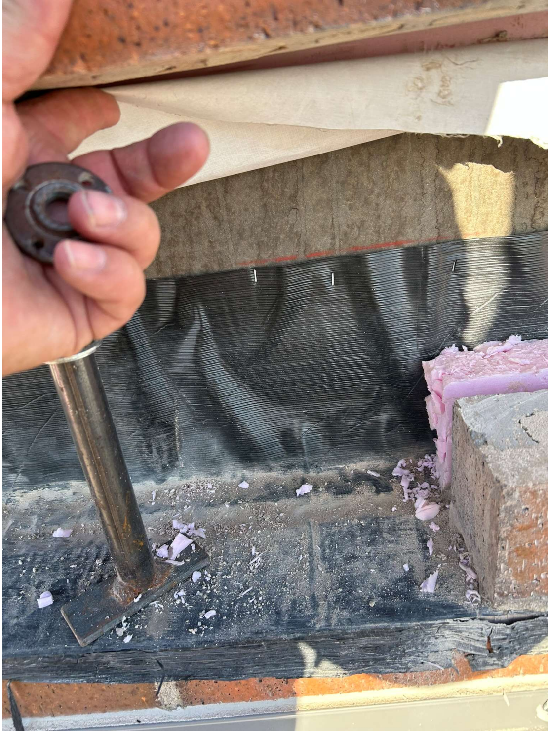
Original through wall flashing detail
