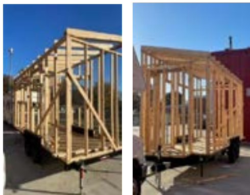
Making Good Progress
