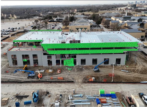
North Elevation – Sheathing, Waterproofing and Glazing Frame Installations
