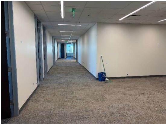
4th Floor – Phase 3 New Offices
