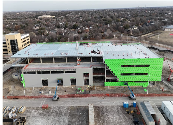
South Elevation – Sheathing and Waterproofing Installations
