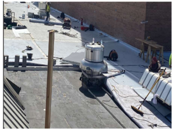
Install of New Section of the Roof
