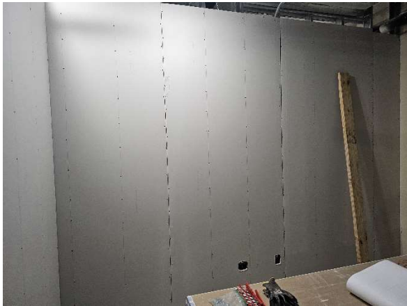
PD – Aux Services 1 Side Drywall
