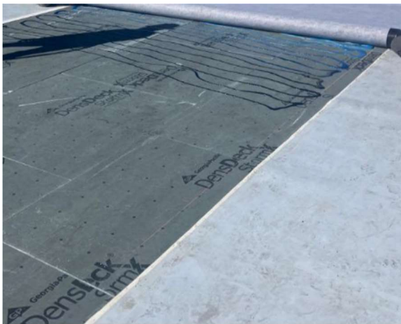
Roof Installation
