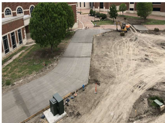
Fire Lane Poured North of Welcome Center
