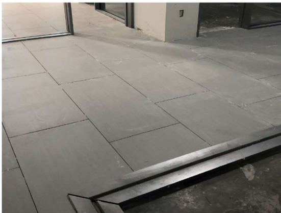
Tile Installed in Veteran's Lounge at Welcome Center
