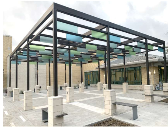
Panels Installed on Trellis at Alumni Hall
