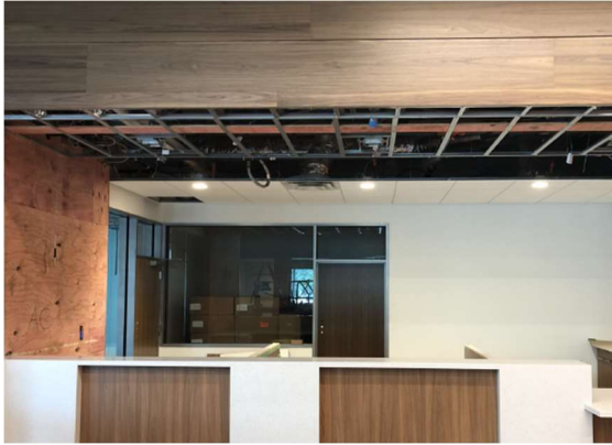
Stone Tops and Wood Ceiling Installed at Transaction Area
