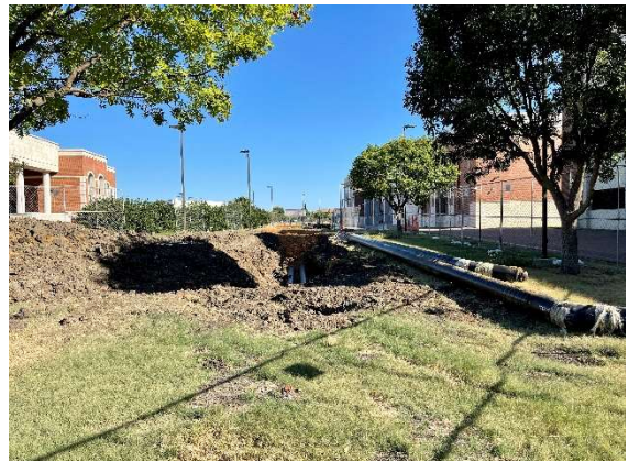
Underground Hydronic Piping Install Behind Library
