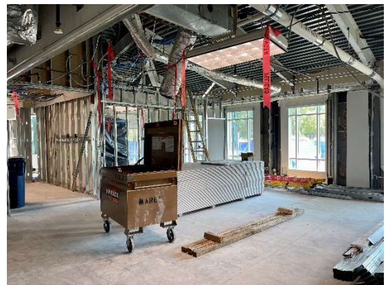
Interior Renovations Founders Hall
