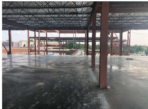
Slab Poured on 2 nd Floor of Welcome Center
