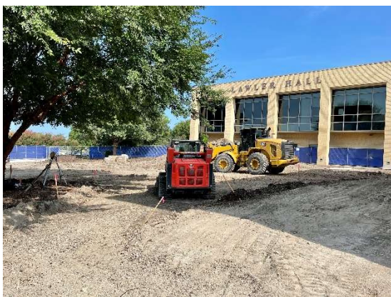
Prepping New Entrance Area for Lawler Hall
