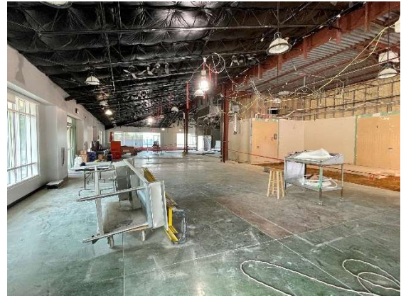
Interior Renovation in Dining Hall
