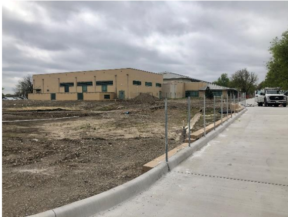
Installation of Guardrails
