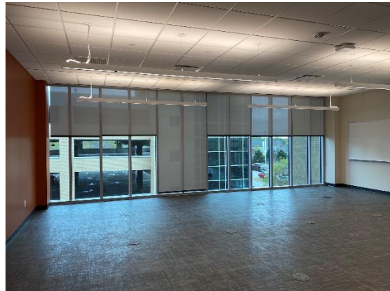
Classroom on 2 nd Floor, NE End
