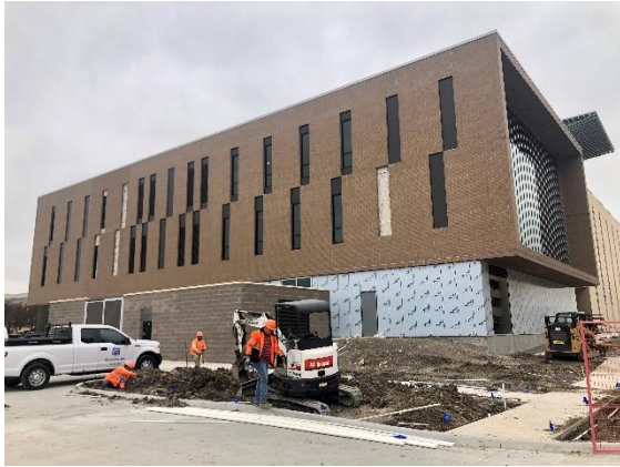
Eastside View of Building
