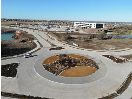
Roundabout at Choate Parkway/Kinship Parkway
