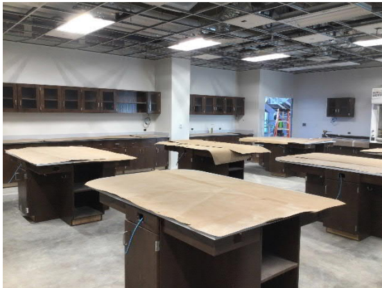
Science Lab Casework Installed
