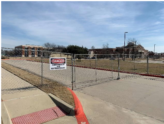
NW View of Fencing Installed for Construction
