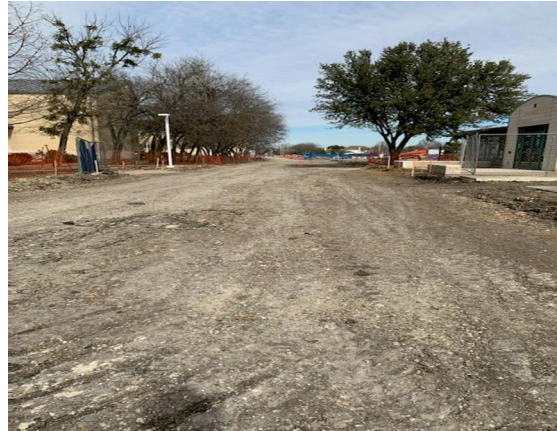
North to South View of Firelane, Ready for Lime Stabilization
