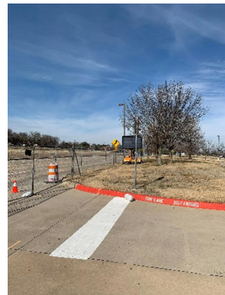
West View of Fencing Installed Along Community Ave
