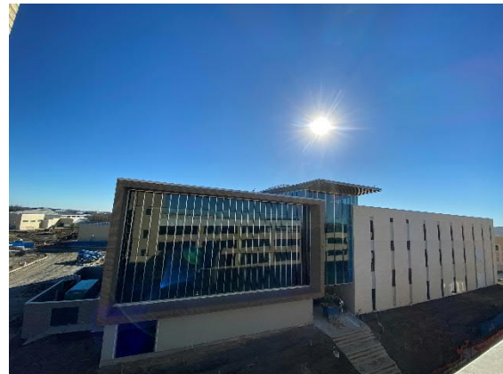
North Curtain Wall
