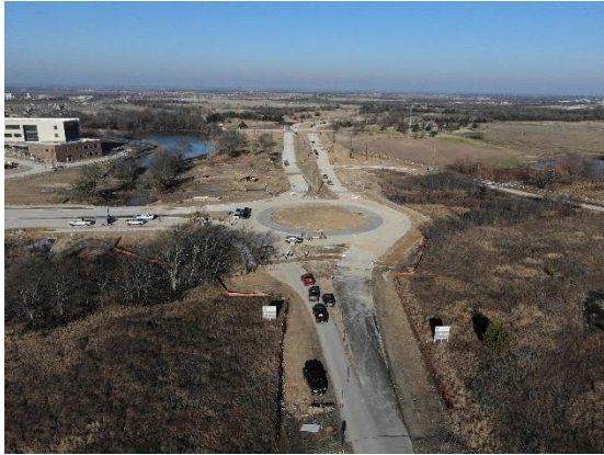
Roadway at West Entrance of Campus
