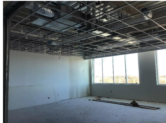
Second Floor Classroom Space in North Building
