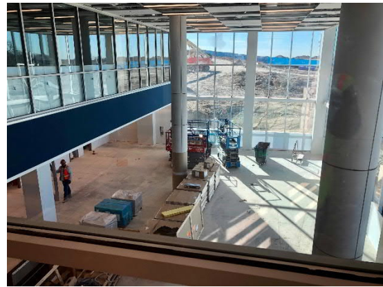
View of Library from 2 nd Floor
