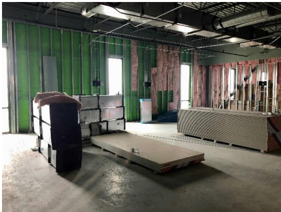
Third Floor Classroom on West side of Building
