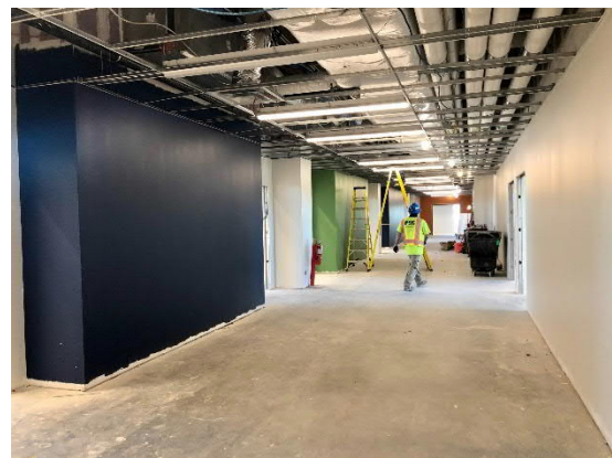
3 rd Floor Hallway in North Building
