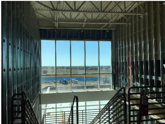
Staircase in South Building
