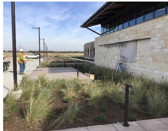
Signage Install at Main Entrance to Building
