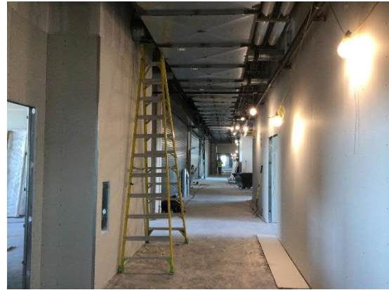
Second Floor Hall in North Building
