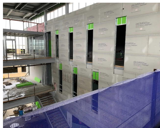
Installation of Atrium Finishes
