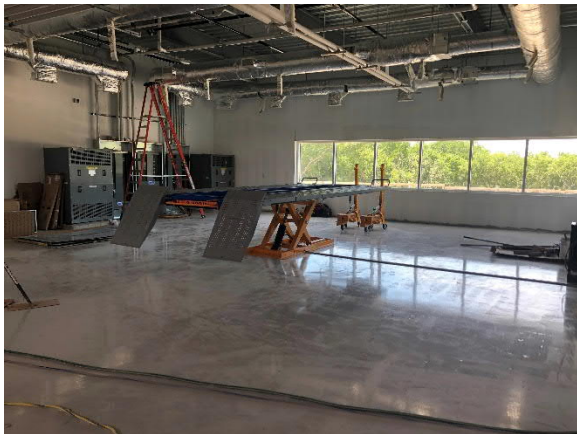
Trade Bar D Car-O-Liner Lift Installed
