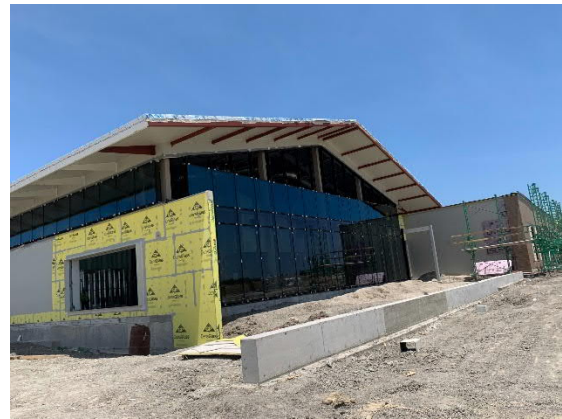
Curtain Wall Install at Library Area
