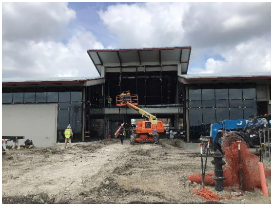
Curtain Wall at Main Entrance
