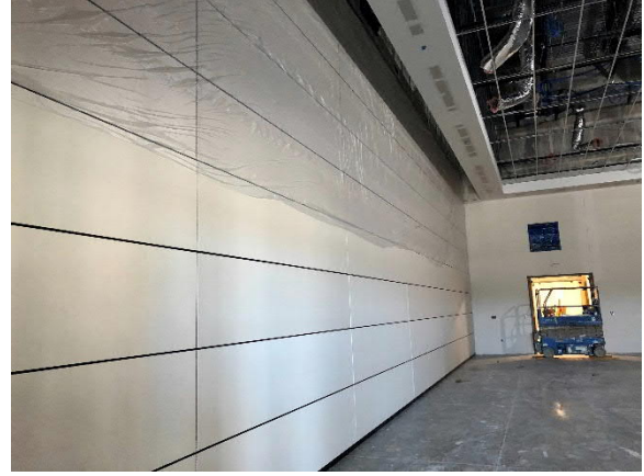
Partition Installed in Conference Center Room
