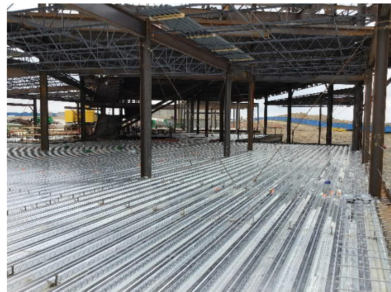
South View of 2 nd Floor of North Building
