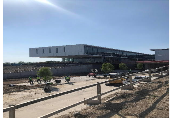
Trees Being Installed at South Garage Entry
