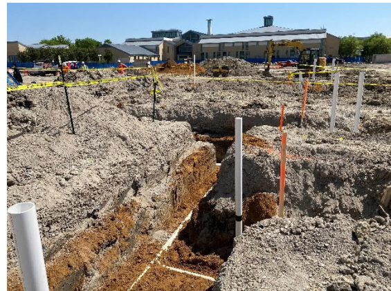
Underground Plumbing Install
