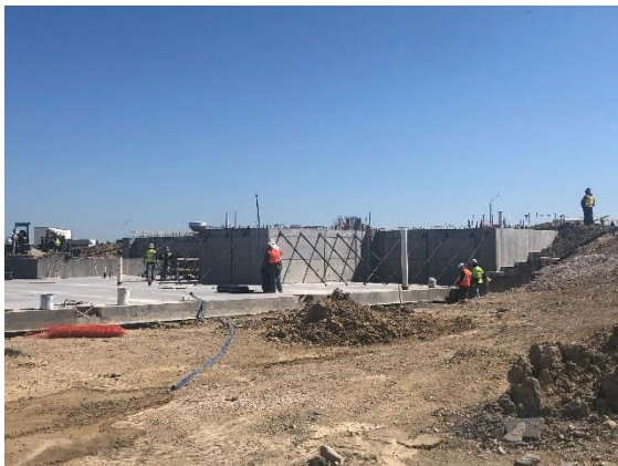
Bracing of South Building Walls
