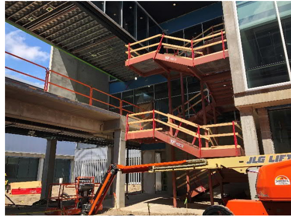
Outdoor Stairs Installed at Trade Bar B
