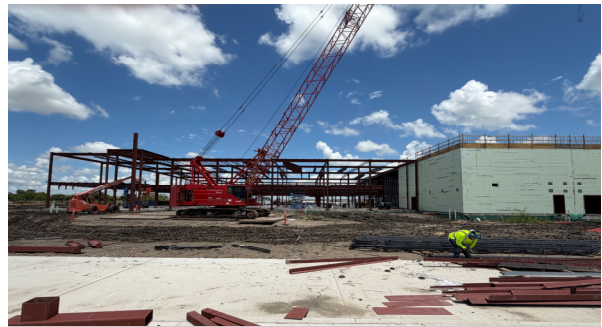
STRUCTURAL STEEL – AREA B CLASSROOMS
