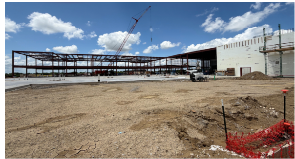
STRUCTURAL STEEL – AREA A CLASSROOMS
