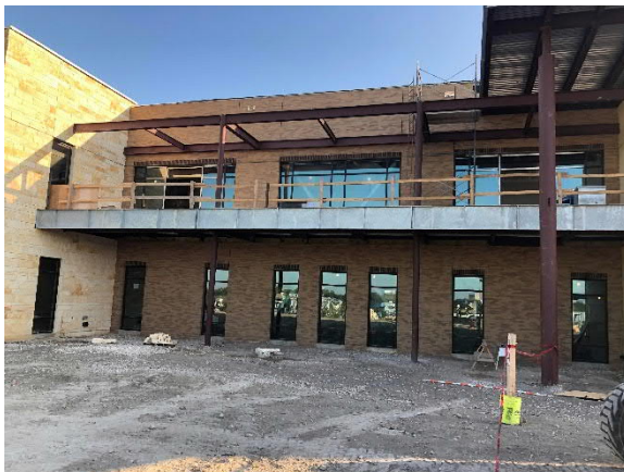
Library – South View of Masonry
