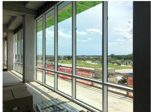
Building A – Window Install
