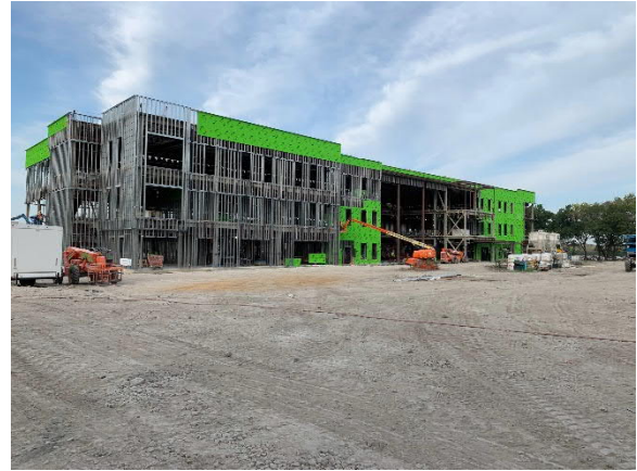
Student Center – North Sheathing
