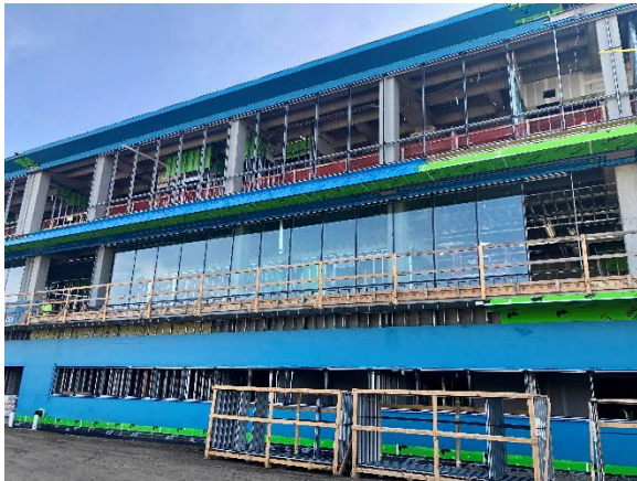
Building A – Window and Eyebrow Install on the West Side
