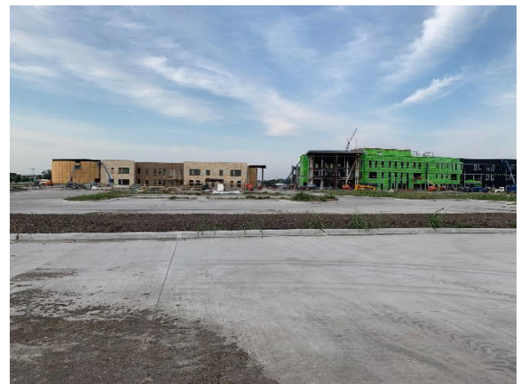
Library and Campus Commons – Exterior View, Facing West
