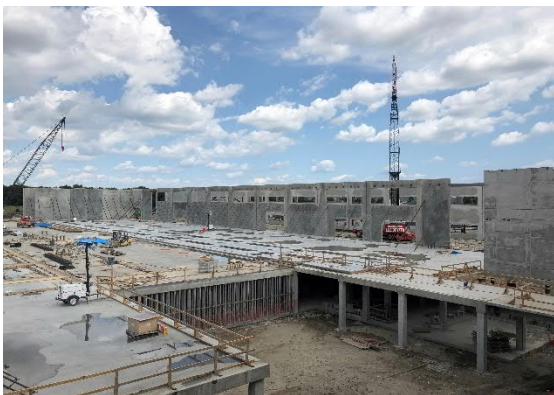
Building C Tilt Erection
