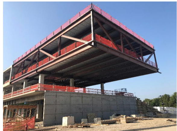
Building A – North Truss
