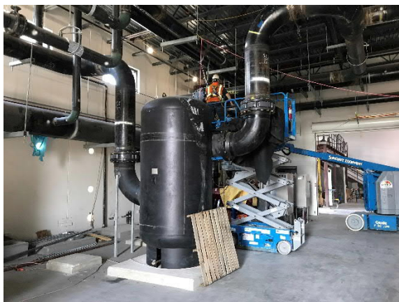
Central Utility Plant – Hydronic Piping Install
