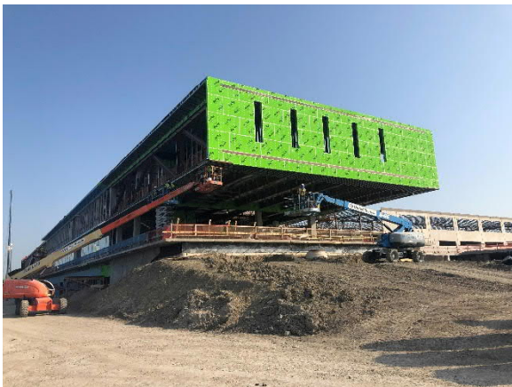
Building A – South Truss
