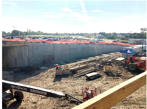
Retaining Wall at South Garage Entrance
