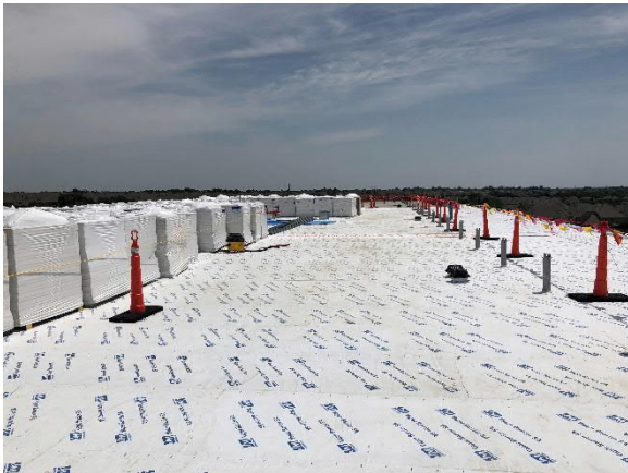
Building A – Waterproofing and Roof Install
