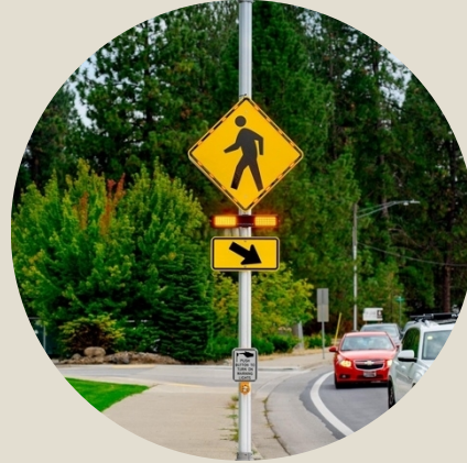
Rectangular Rapid Flashing Beacons (RRFBs)
