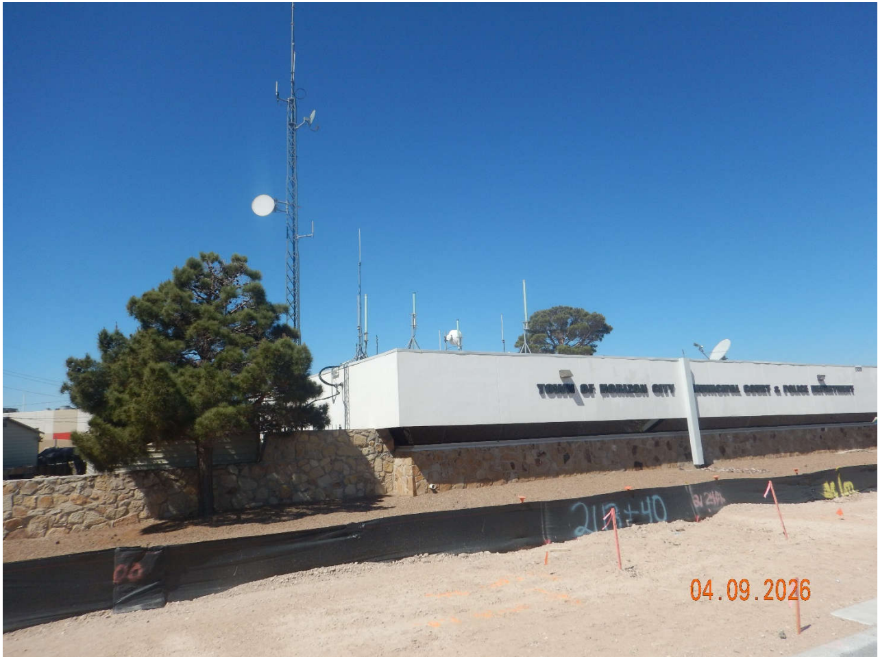
Photo showing existing self-support tower and roof-mounted communications equipment.
