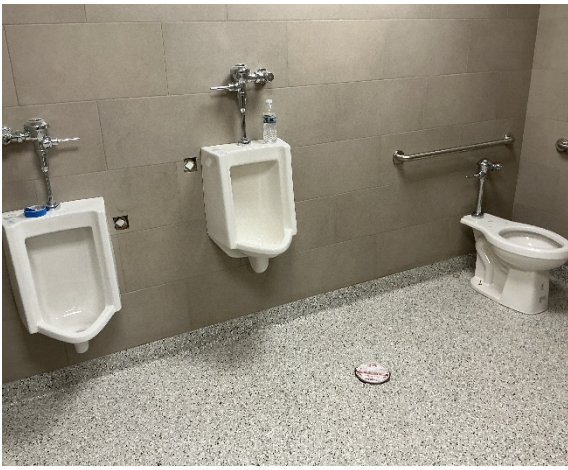
MEP finishes continue throughout the site
