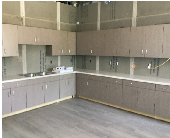
Casework installation on the 1 st floor
