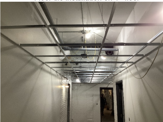
Ceiling grid installation in the basement
