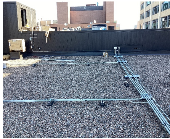
Mechanical unit rough-ins continue on the roof
