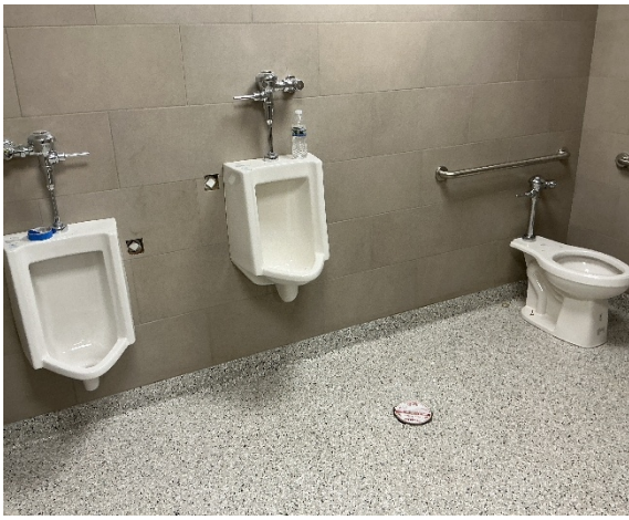
MEP finishes continue throughout the site
