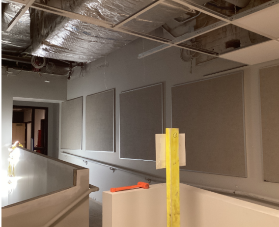
Tack Boards through the ramp
