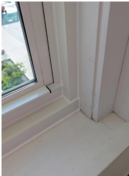
Caulking at Windows
