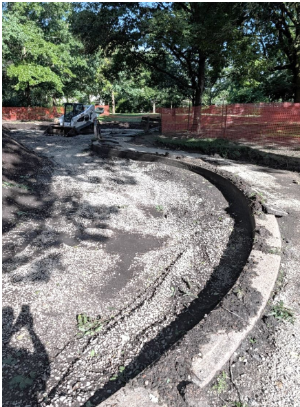
Existing Concrete Curb Demolished & Removed
