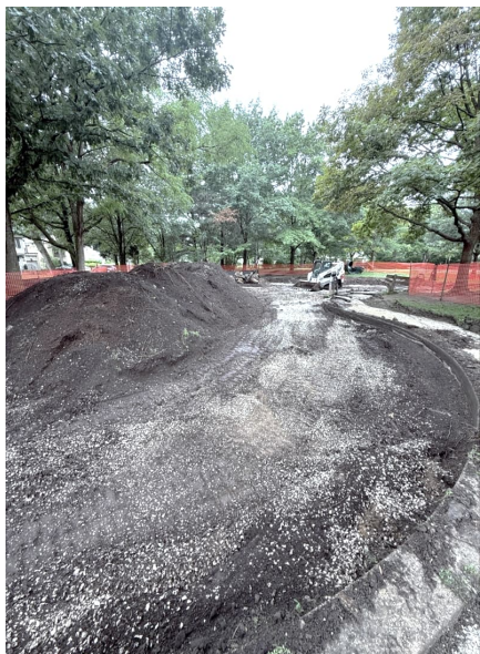
Existing Concrete Curb Demolished & Removed
