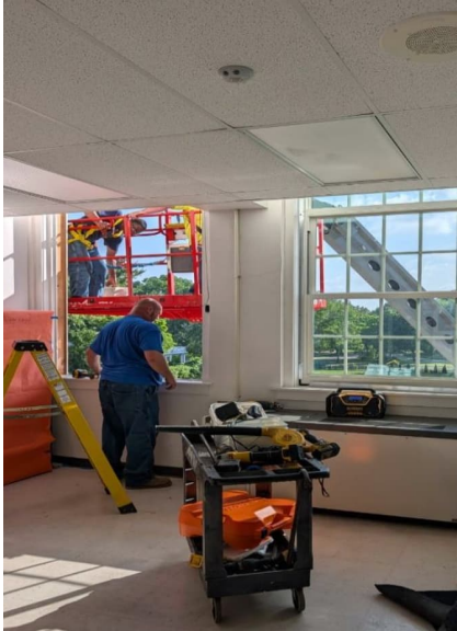
Windows Installation In Progress
