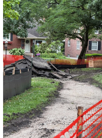
Existing Asphalt Removed
