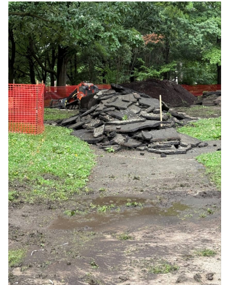
Existing Asphalt Removed
