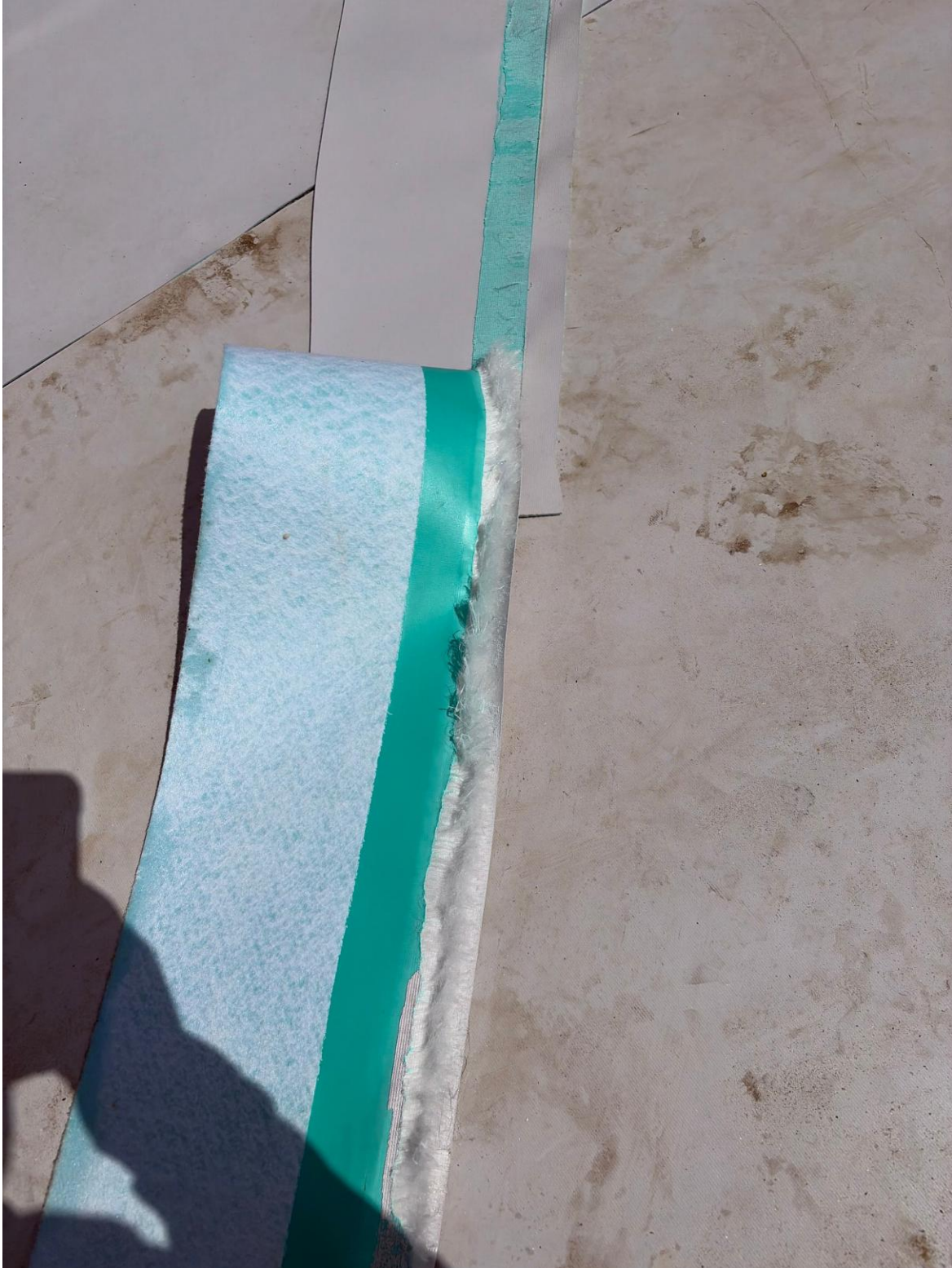
Daily weld test
