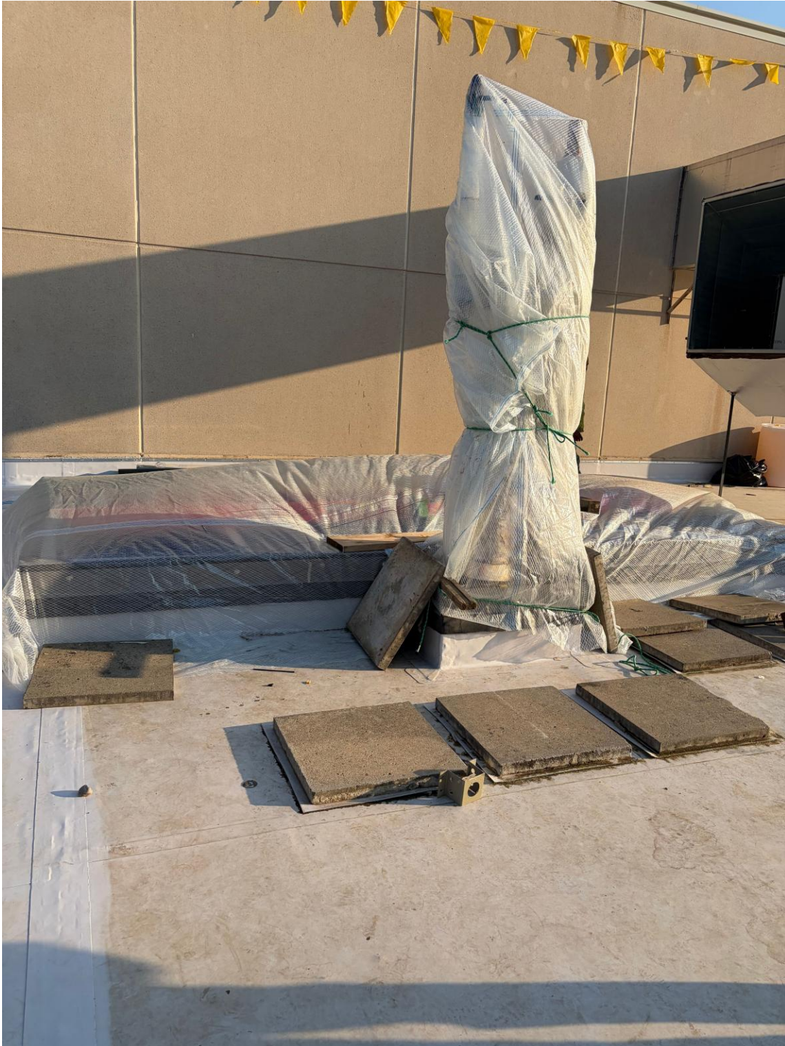
Unit removal: Tied off open roof area prior to storm on roof area #5
