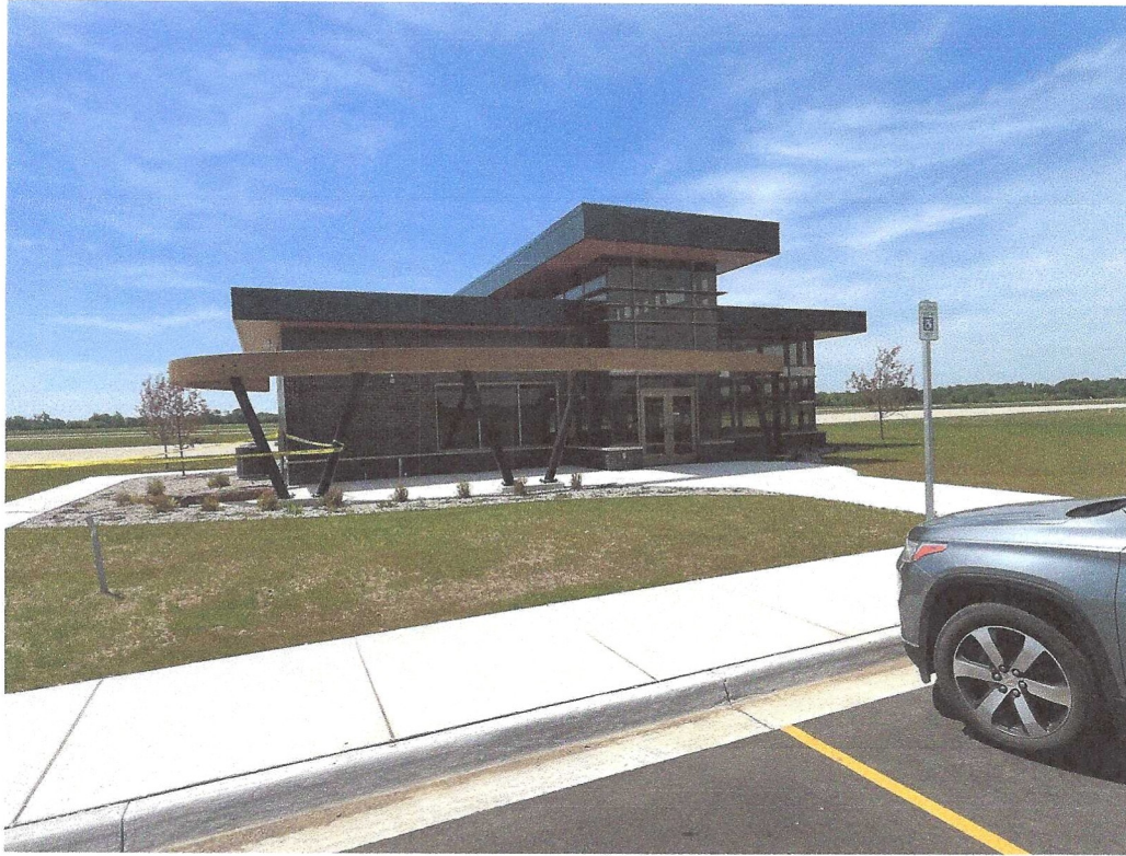
June 04, 2026 - Hillsdale Terminal
