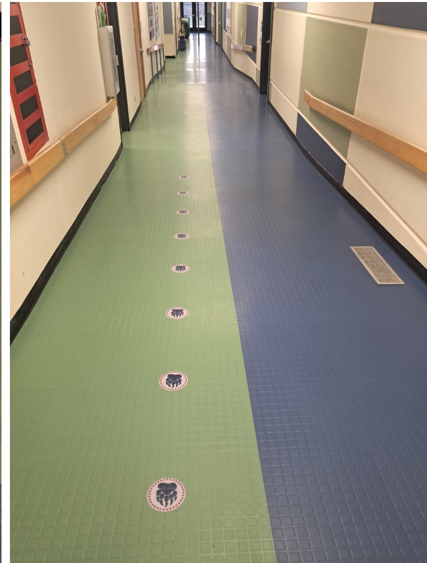
Y.V. Finished non-slip floor
