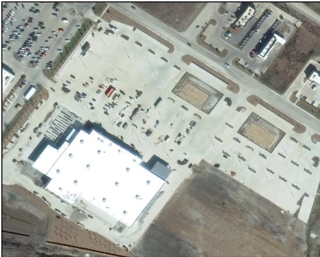
Lowe's construction as of February 2026
